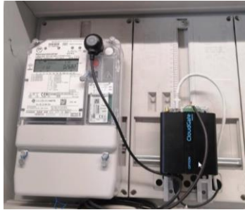
Figure 2: Test version / 1st test bed Druckerei Roser, Salzburg using load profile meter and the optical interface – no scalable version
